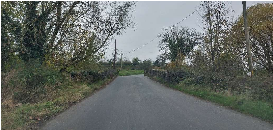
Plate 13.27: Grid Connection Route crossing Brittas Bridge (BH25), facing west
