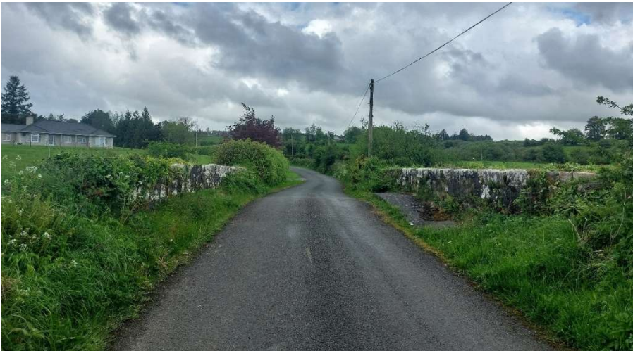
Plate 13.15: Grid Connection Route crossing Scarrough Bridge (BH5), facing north
