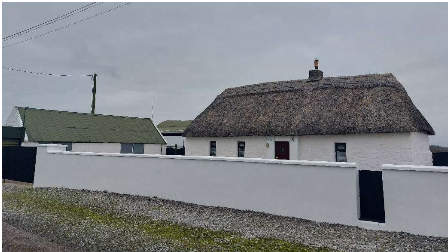
Plate 13.30: Grid Connection Route passing thatched cottage (BH26) in Killinure, facing northwest
