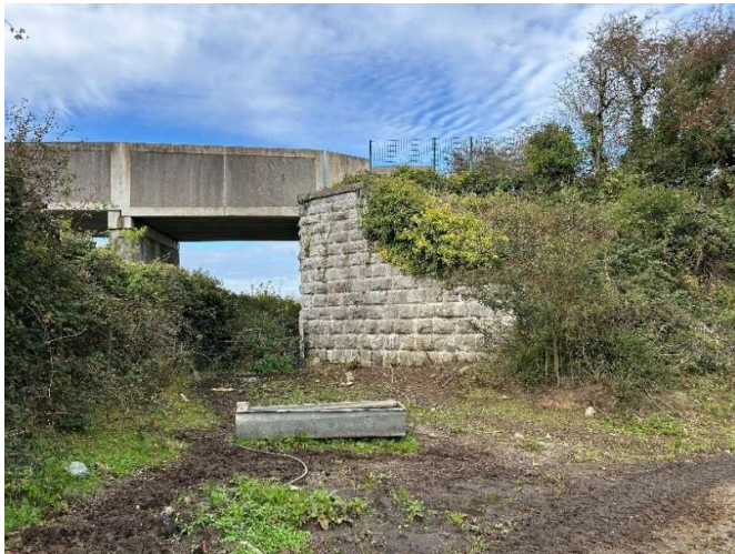
Plate 13.36: Proposed Grid Connection Route, where it passes beneath the railway line (showing railway bridge CH130), facing northwest
