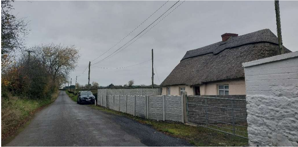
Plate 13.29 Grid Connection Route passing thatched cottage (BH26) in Gorteenaskagh, facing northwest
