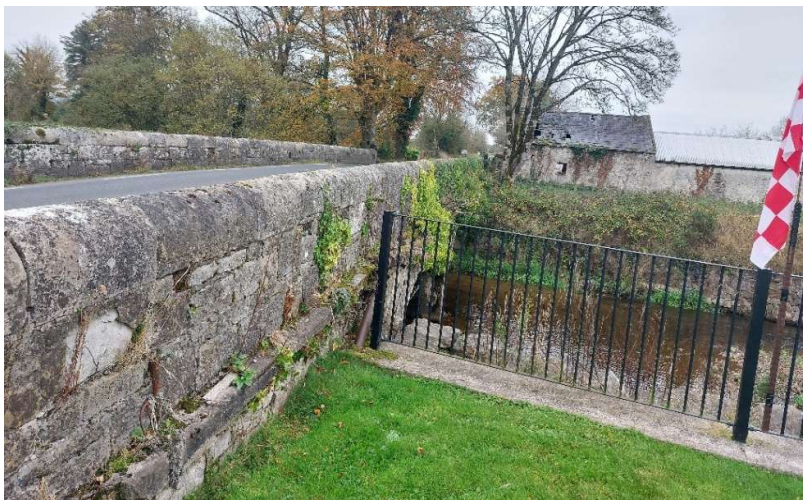
Plate 13.25: Grid Connection Route crossing Cappamore Bridge (BH23), facing east
