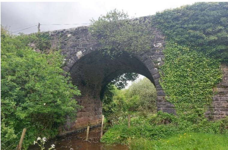
Plate 13.16: Western façade of Scarrough Bridge (BH5), facing northeast
